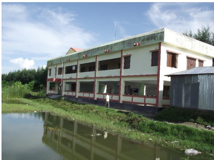
A cyclone shelter with open ground floor
