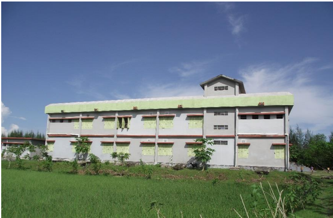
Cyclone shelter on Noler char
