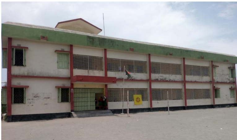
A cyclone shelter with enclosed ground floor
