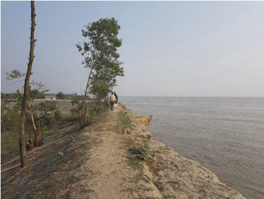
Fig. 3.1. Riverbank erosion in Shantipur, Noler Char, 2018.
