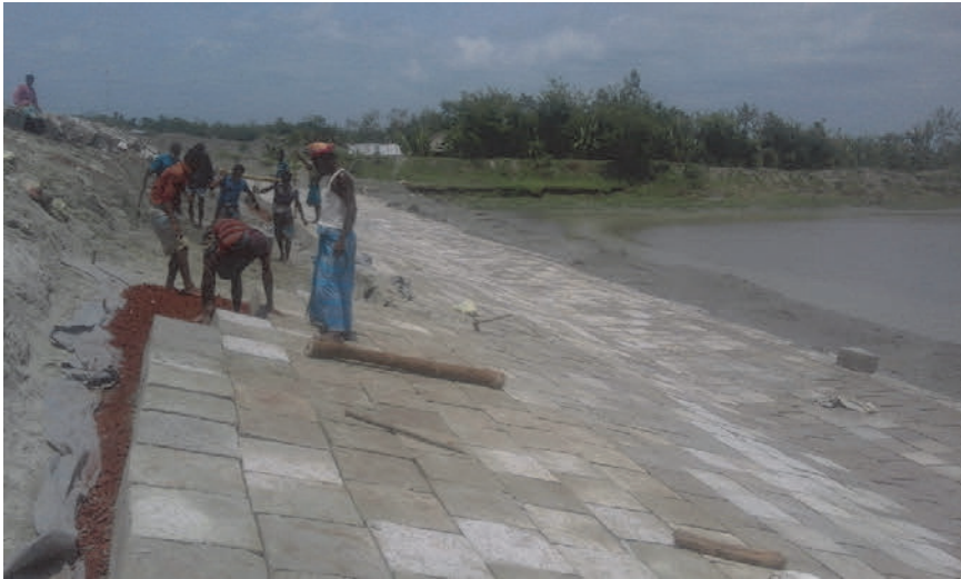
Fig. 6.2. Construction of Caring khal closure, Char Nangulia.
