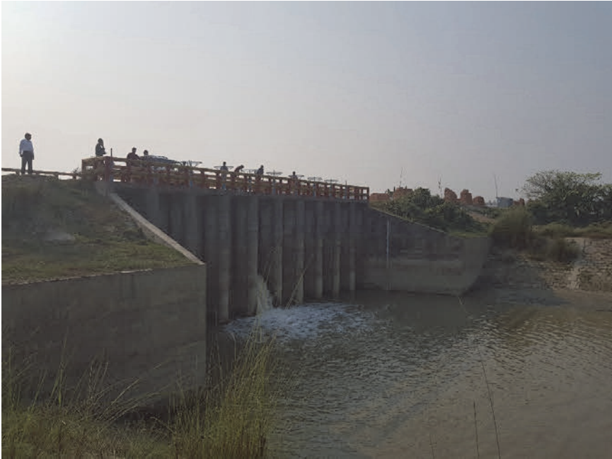
Fig. 6.1. Drainage sluice, Char Nangulia.
