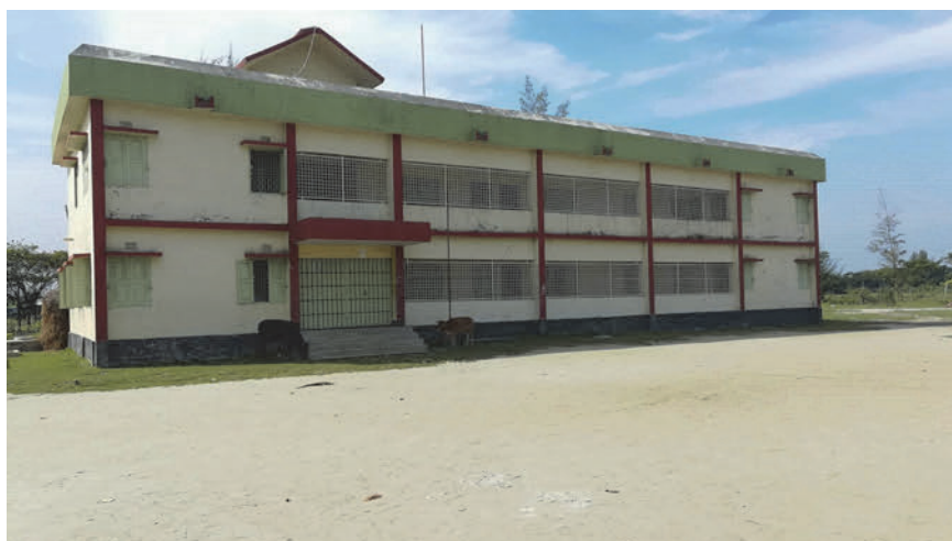
Fig. 6.5. Thanarhat Bazar Multipurpose Cyclone Shelter cum Primary School, Noler Char.
